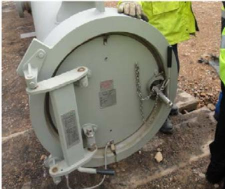
Premtech Ltd manages infrastructure projects in the Energy sector and was asked by National Grid to look at the unpredictable failure the integrity of its transmission network of pig trap door seals and the fitness for purpose of the seals currently in use. BHR Group undertook a desk study on behalf of Premtech as part of this project.
